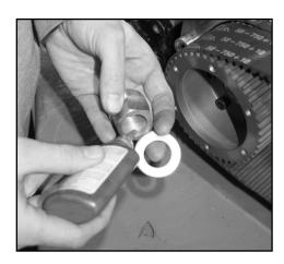
**3.** Install the motor pulley nut using RED Loctite and Torque to Mfg recommended Specification.
